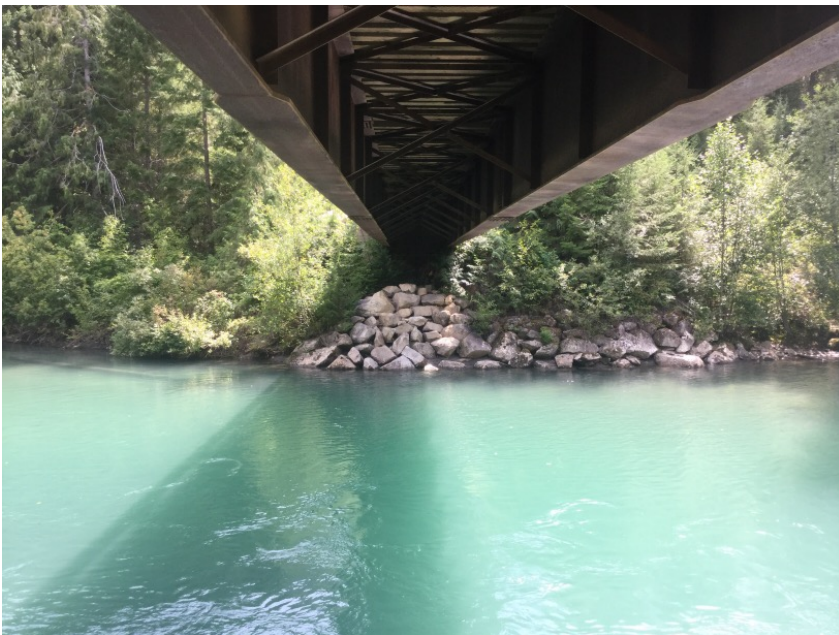
Right Bank Abutment
