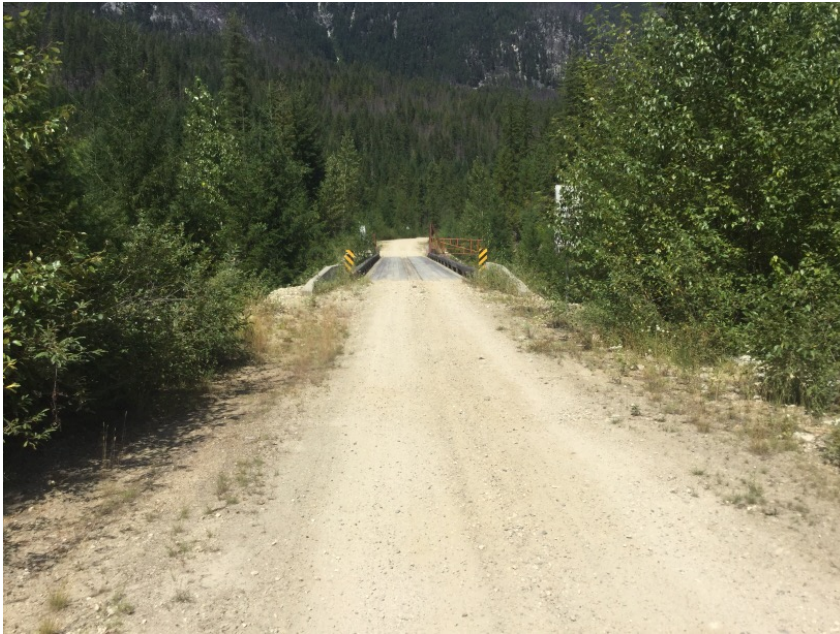
Right Approach Facing Bridge
