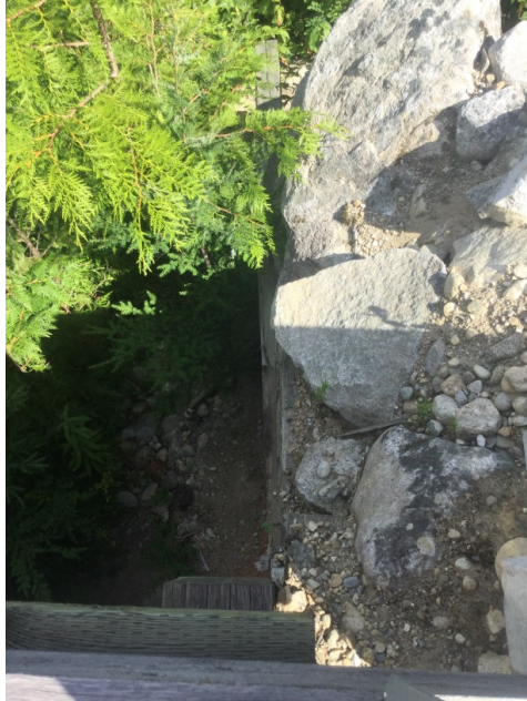
Right Bank Downstream Ballast Wall
