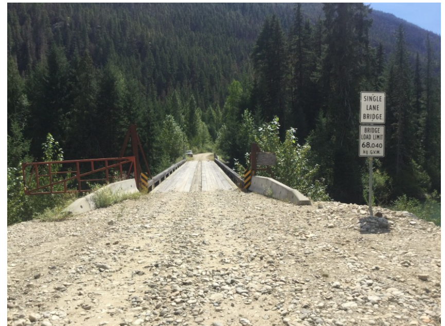
Left Approach Facing Bridge
