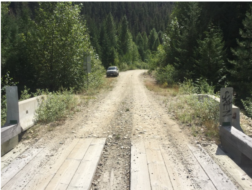
Right Approach Facing Away From Bridge
