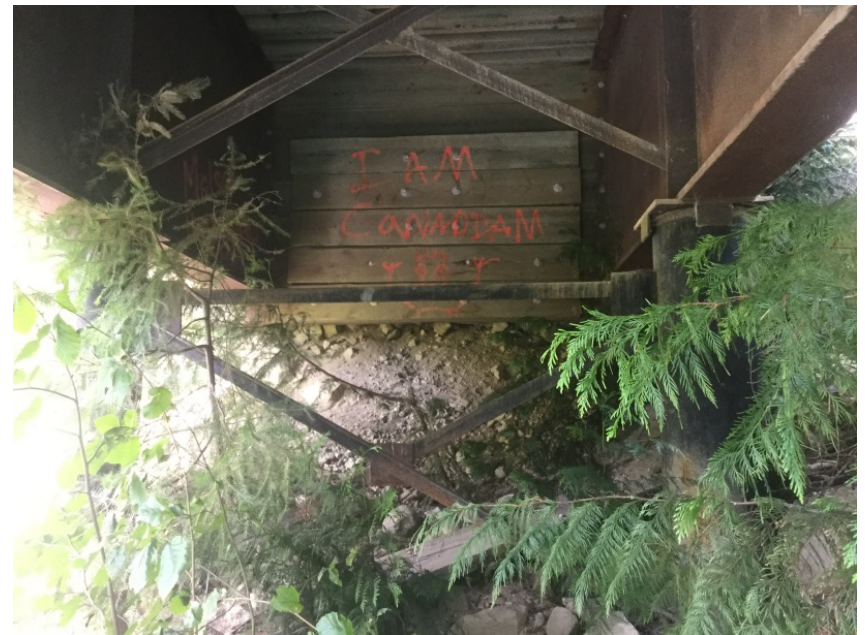
Left Bank Abutment
