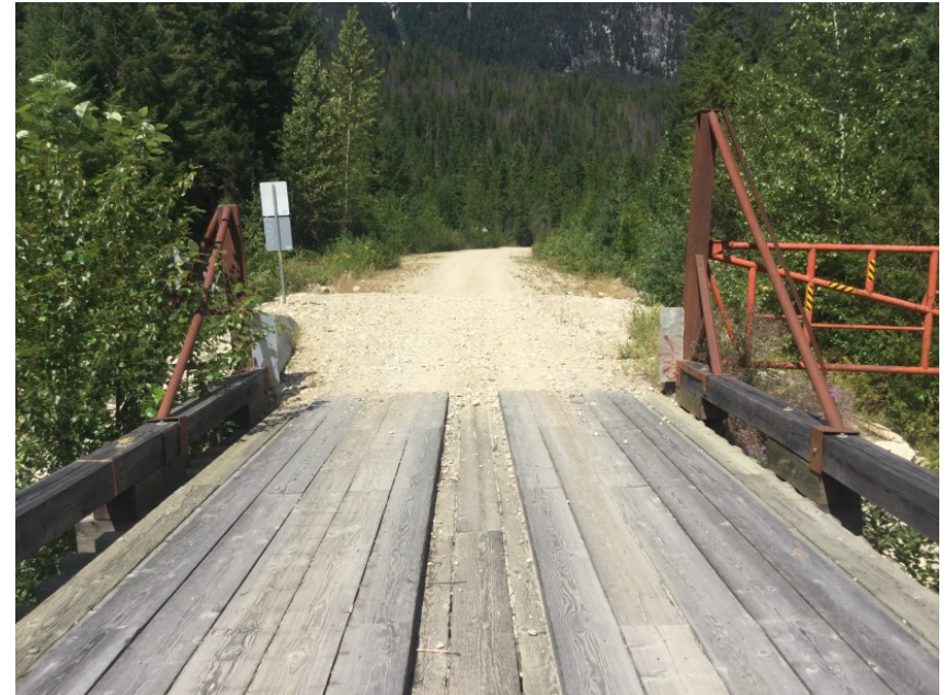
Left Approach Facing Away From Bridge
