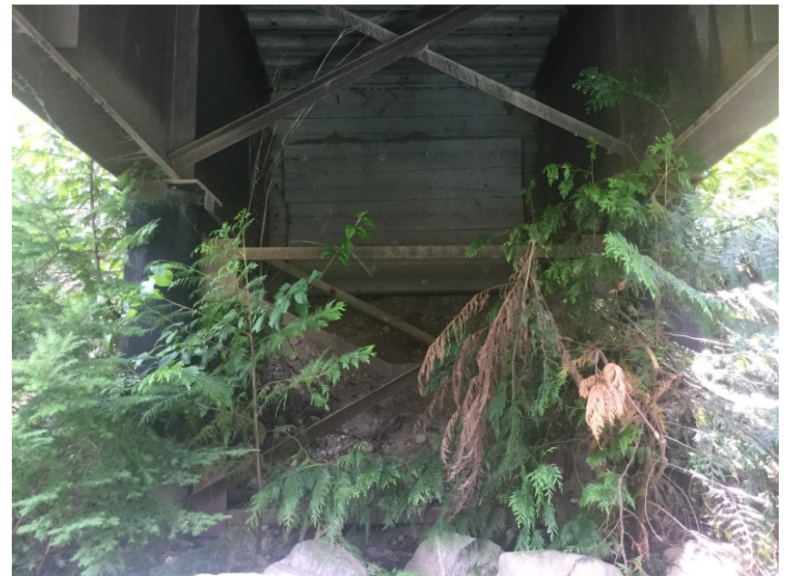
Right Bank Abutment
