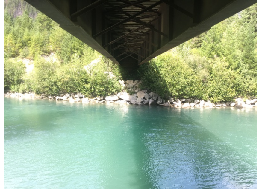
Left Bank Abutment
